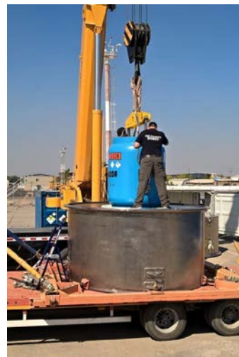
Fig. 21. Mounting of TUK-145/C package
