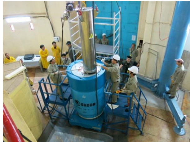
Fig. 7. Reloading of FA from the transfer cask, Vietnam
